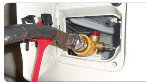
CNG Filling Equipment
